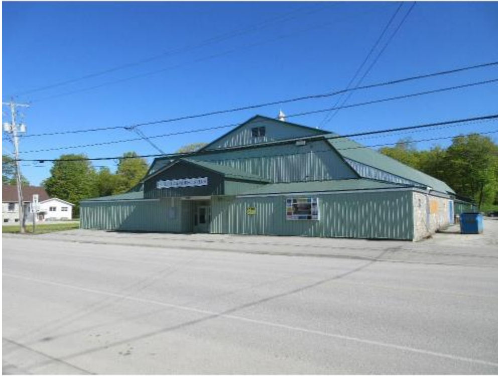
Photo 1 – Exterior of Mindemoya Arena. Front entrance along highway 542
