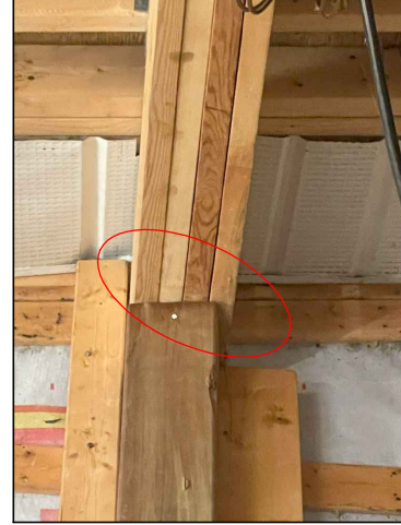
PHOTO 4 4-PLY BEAM OVER-HANGING WOOD COLUMN
