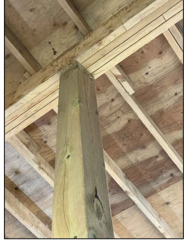
PHOTO 2 TYPICAL WOOD COLUMN TO BEAM CONNECTION
