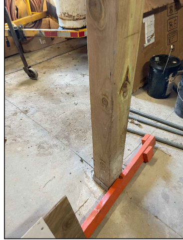
PHOTO 1 TYPICAL WOOD COLUMN
